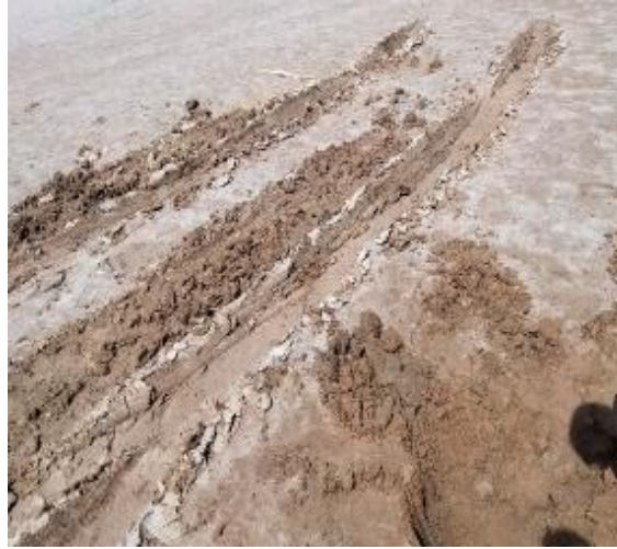
Fig 3-10. Damage caused on Sebkha surface by track's wheels.
