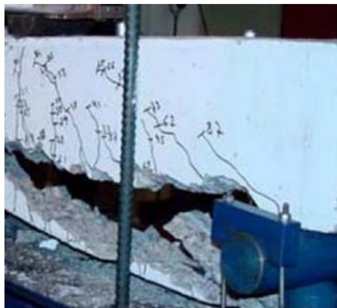
Figure. 1.13 Bar-end cover separation failure mode [79]
