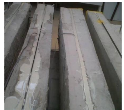
c) groove cutting, placing of CFRP bars and epoxy filling
