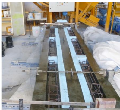
a) Steel reinforcements assembling
