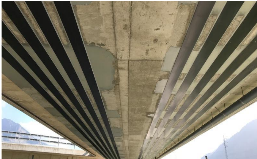
Figure 1.6 Externally Bonded Reinforcement (EBR) [51]
