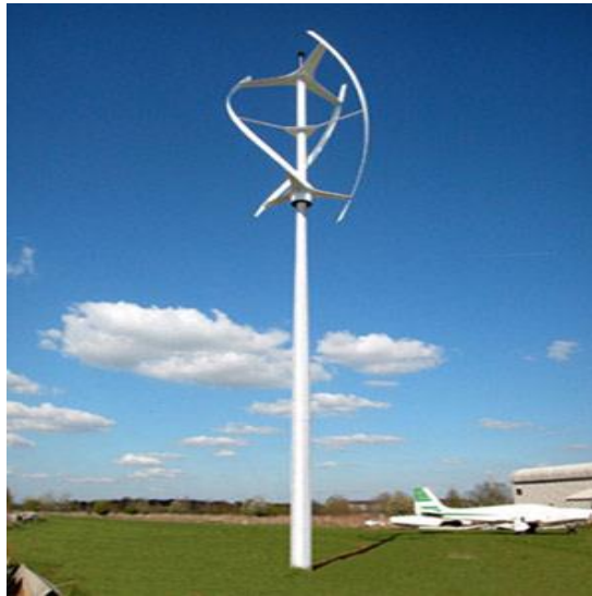
Figure 5.2 Darrieus type vertical axis wind turbine
