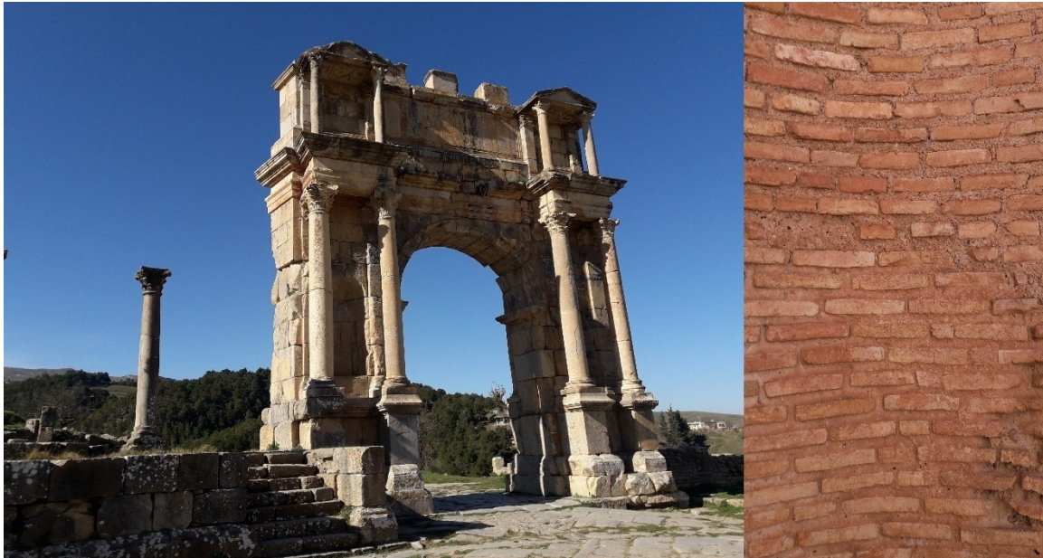
Fig.IV.8: The Caracalla arch and the separation wall of the dated brick
