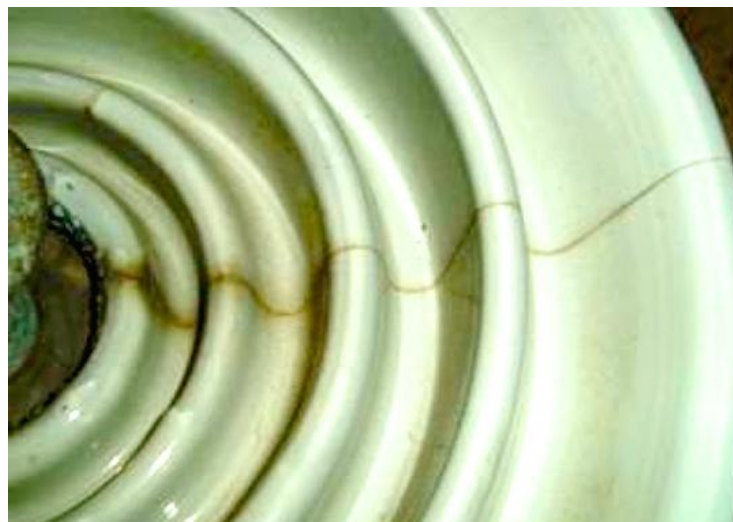
Figure 2. 3 Radial cracking due to cement growth on porcelain insulators [2.6].
