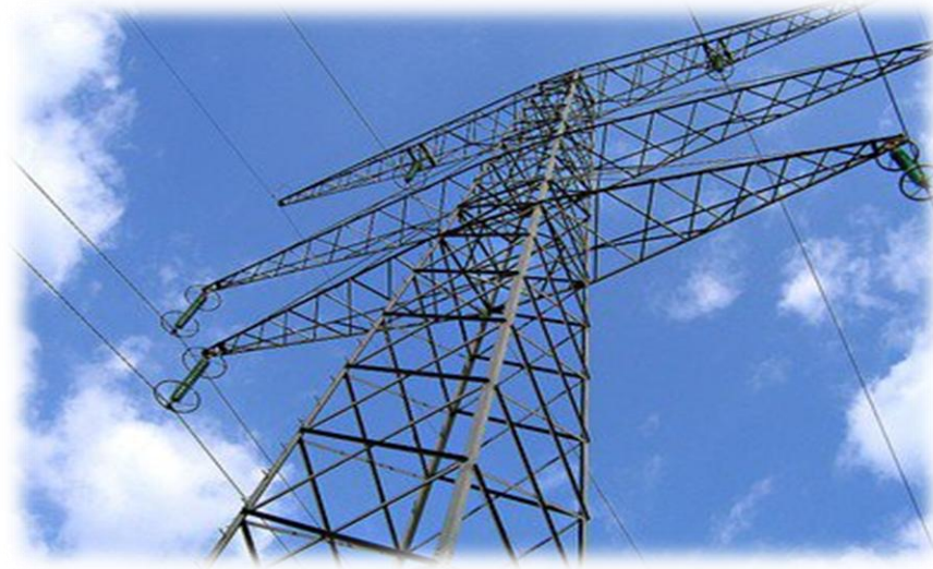
Figure 3. 1 Insulator string equipped with corona rings
