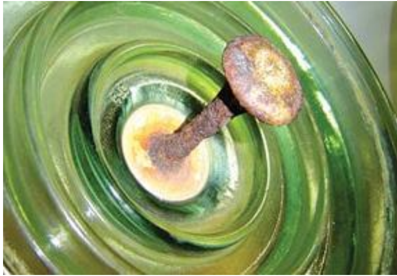
Figure 2. 4 Corroded pin in porcelain insulator
