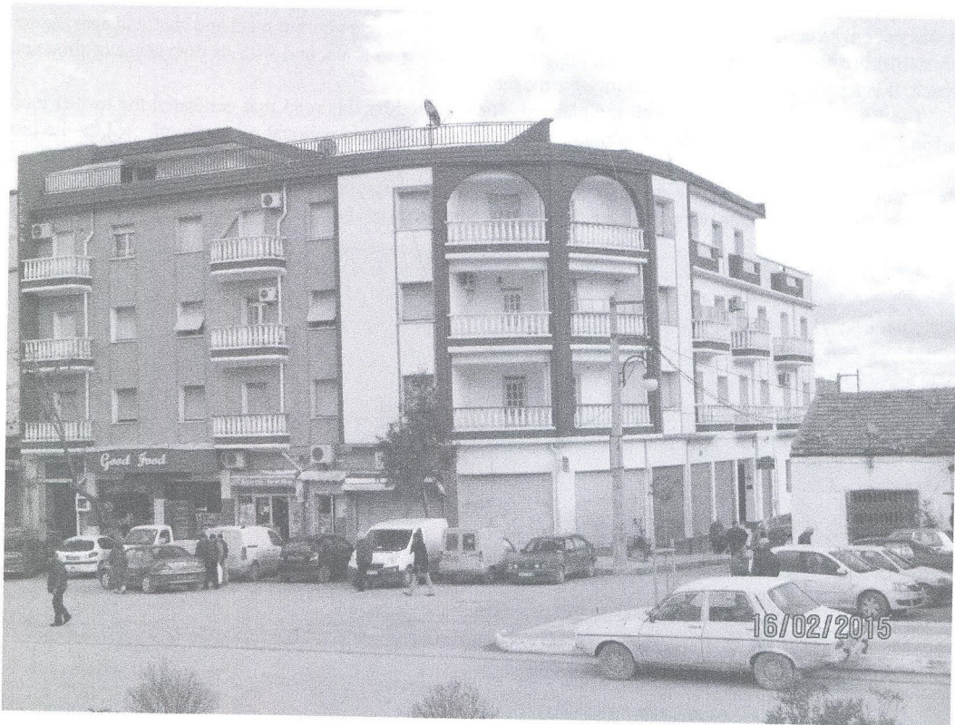
Figure 9.2 In the main street of Ain Arnat all ground-floor plots are occupied by commercial activities
