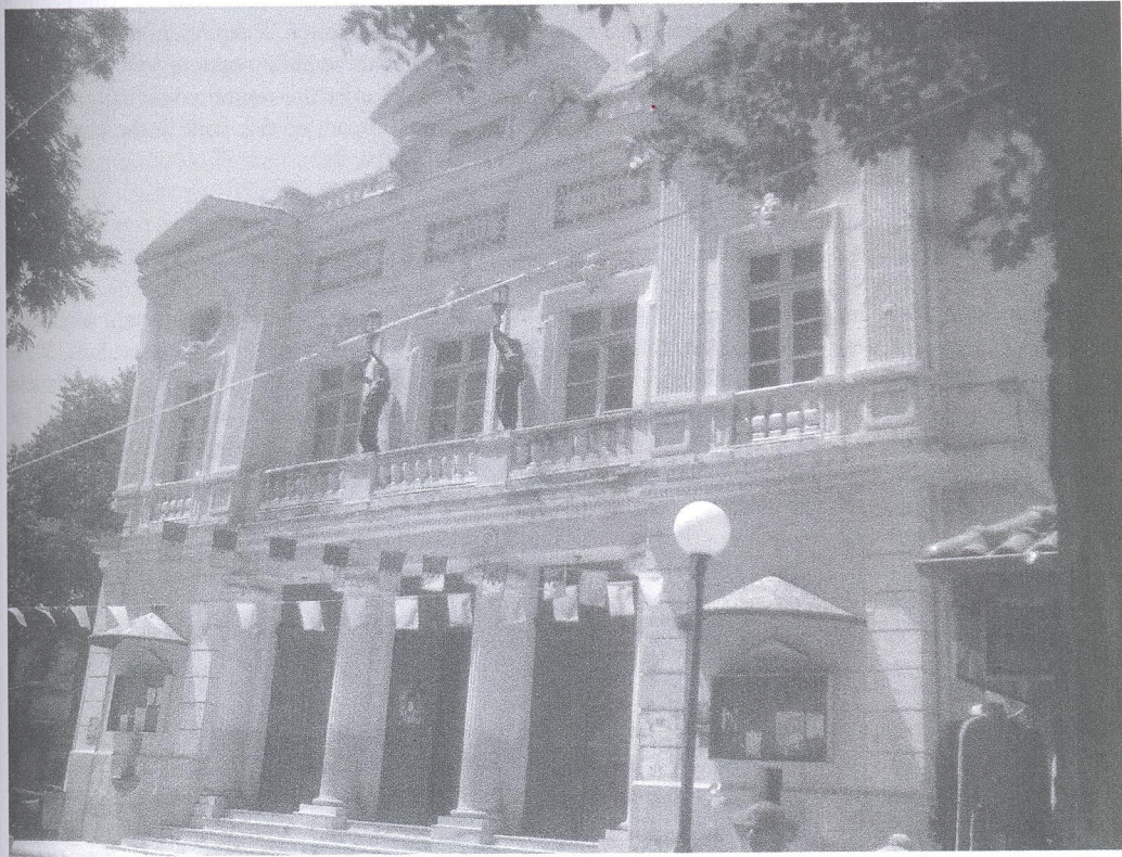
Figure 8.1 The municipal theatre of Setif after the 1990s rehabilitation works
