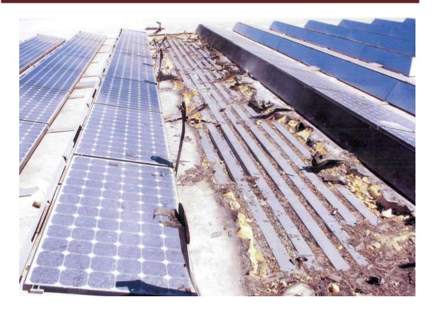
Figure 1.2: Fire hazards in a 383kW PV array, in Bakersfield, California, in 2009 [1.6].
