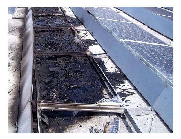
Figure 1.1: Fire hazards in a 1,208kW PV array, in Mount Holly, North Carolina, in 2011 [1.9].
